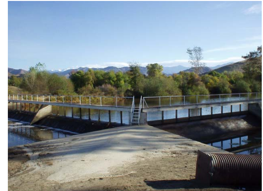
McKay's Point Water Control Facility
