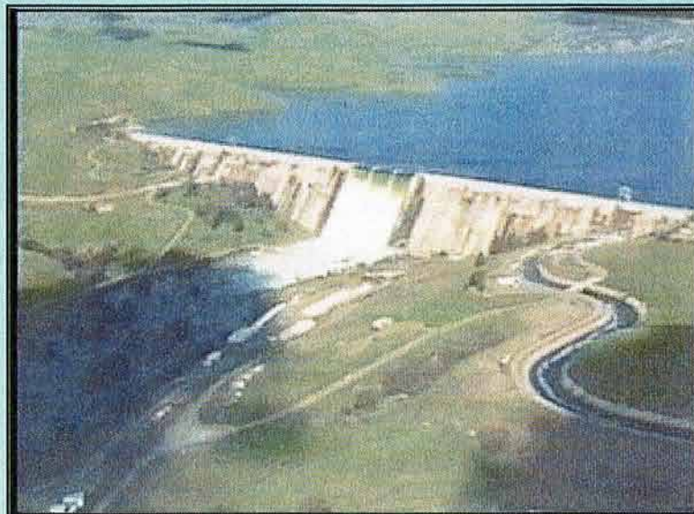
A Millerton Lake spill like the one pictured at left was avoided in part by the quick acting and hard work of the employees of TID, other Friant districts, and the Friant Dam operators. This aerial photo was taken in 2006.
