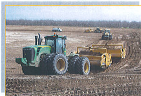
TID Crew constructing Swall Basin—March 2011
