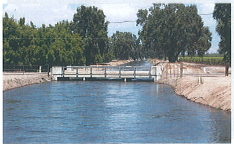
Main Intake Canal as it enters Tulare Irrigation District
