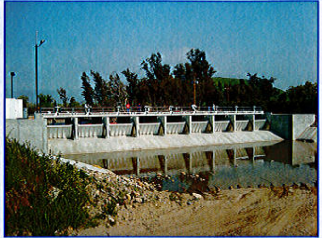
New structure on the Lower Kaweah side, with gates installed
